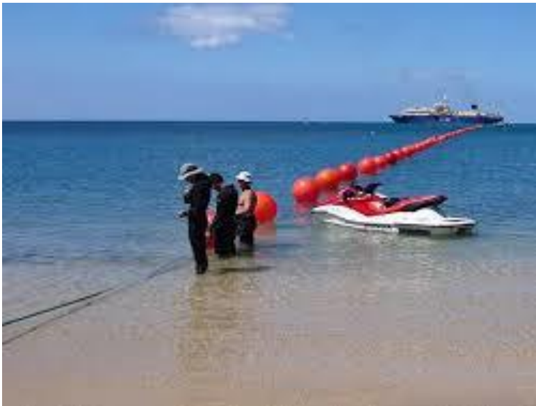
Shore Ends Installation
