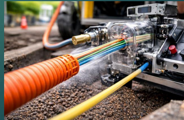
Fiber Cable Blowing
